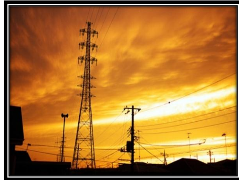
Picture 10 Bulk Supply Electricity Lines
