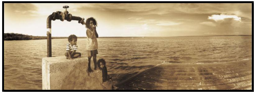
Picture 13 Bulk Water Reservoir
